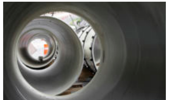
Testing of the interior coating of pipes during pipe manufacturing
