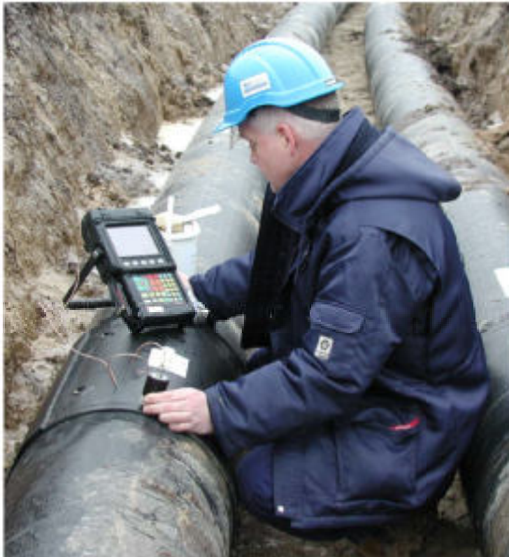
Ultrasound examination of electro-welded district heating mantles
