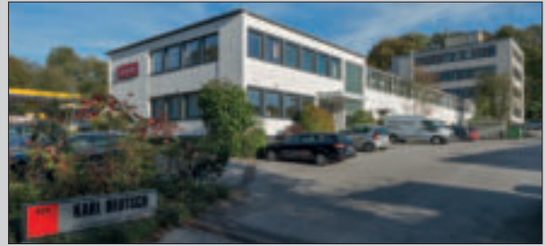
Works 1 was erected in 1967 and extended in 1972. Administration and the sales department are headquartered here. Portable test instruments, sensors and chemical test liquids are produced in Works 1.
