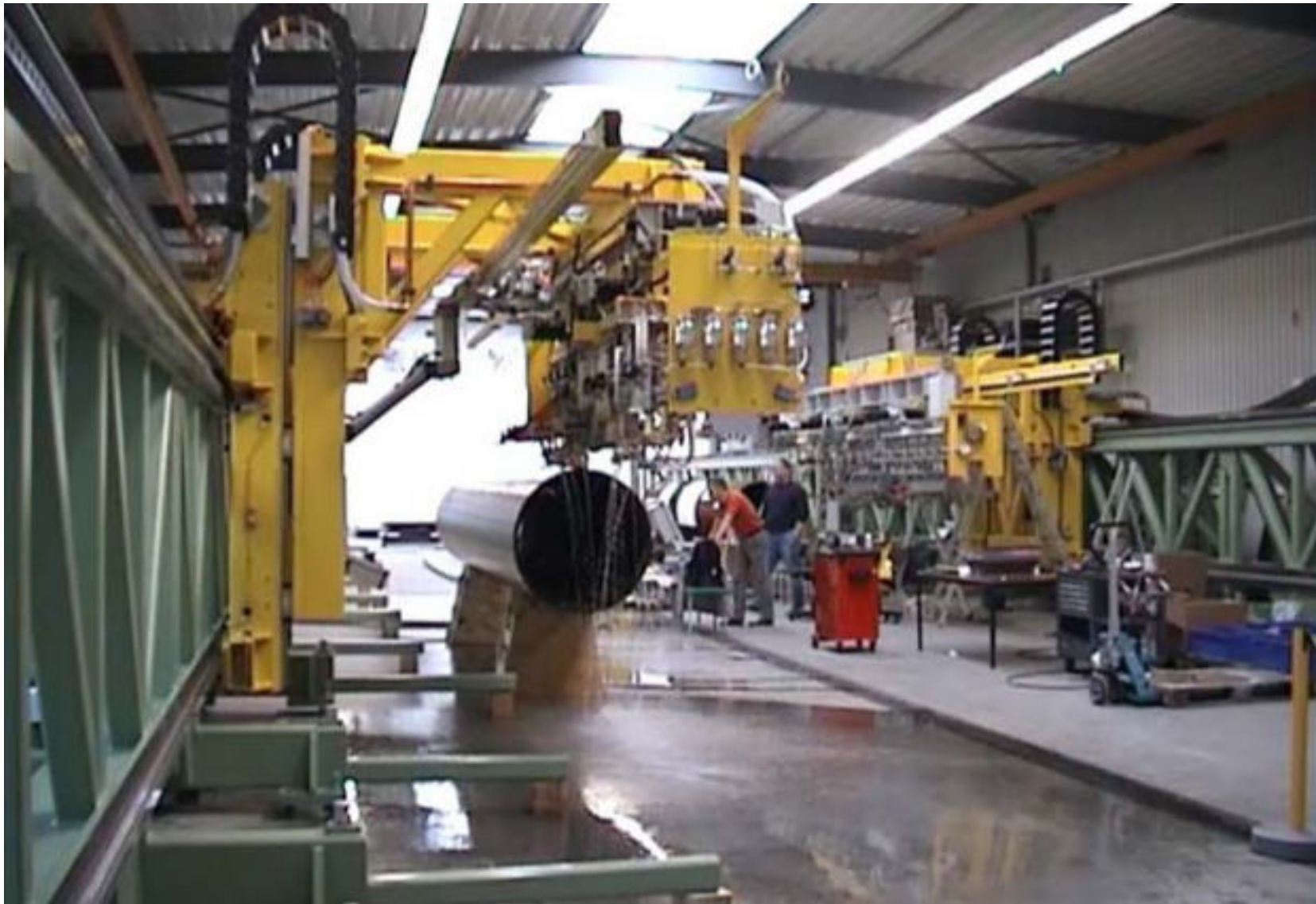
SNUL Prüfportal (2 Stk) Testing Portal (2 systems) @ BAOSTEEL 2007
