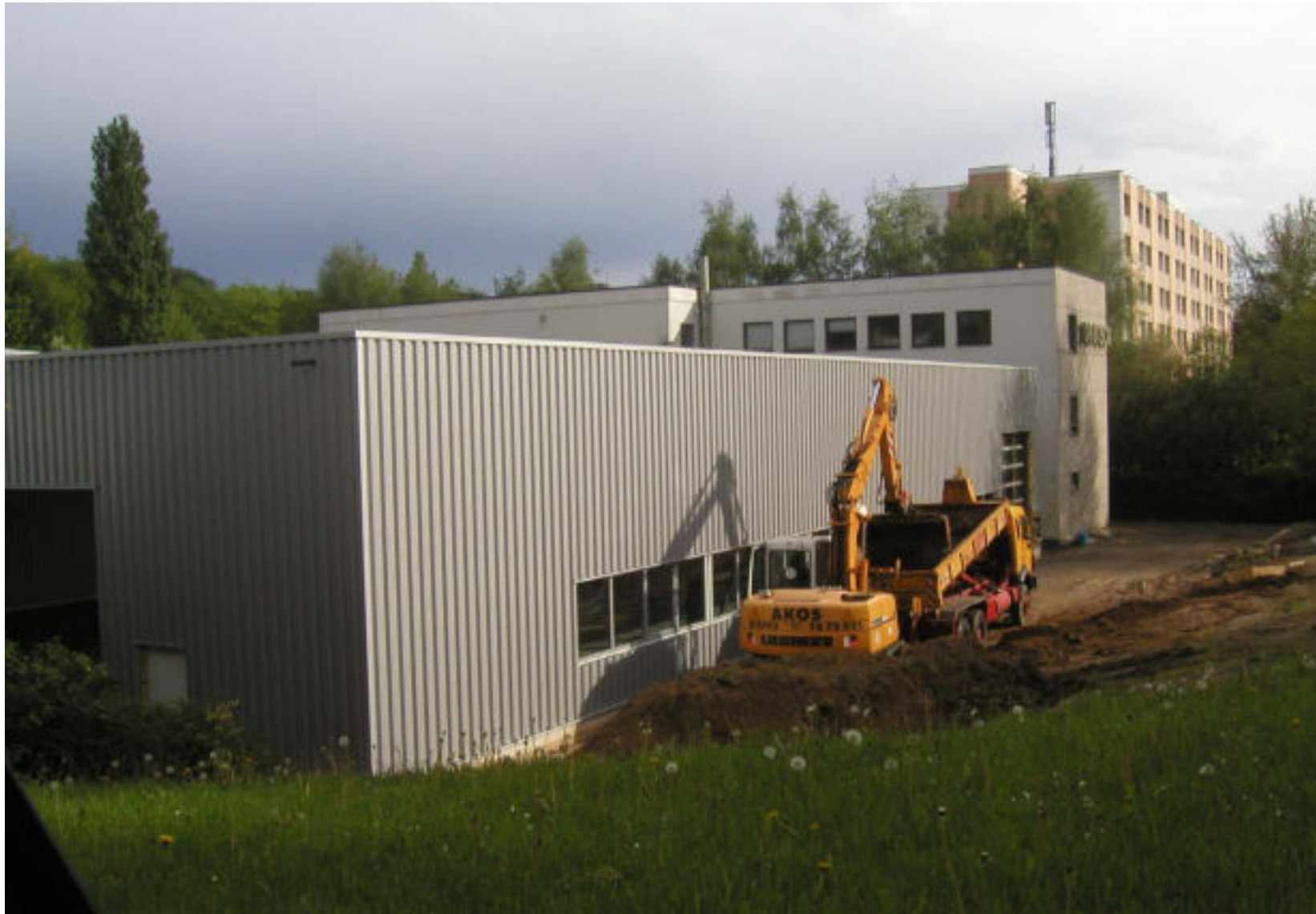
Werk 2 Hallenanbau Works 2 Extension (During Construction)
