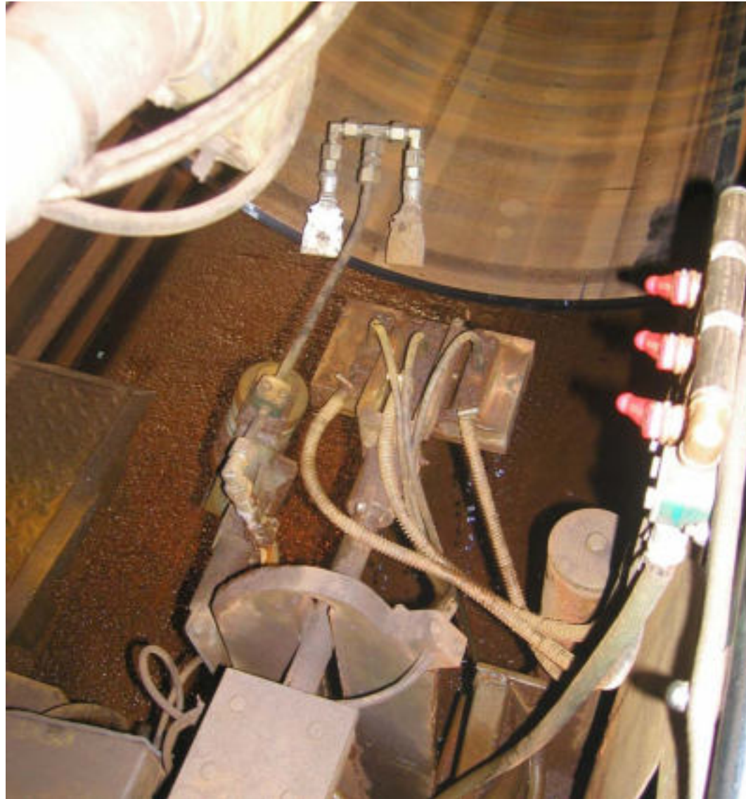
Rohrenden-Prüfung (von innen) LSAW-Pipe End (from internal pipe surface)
